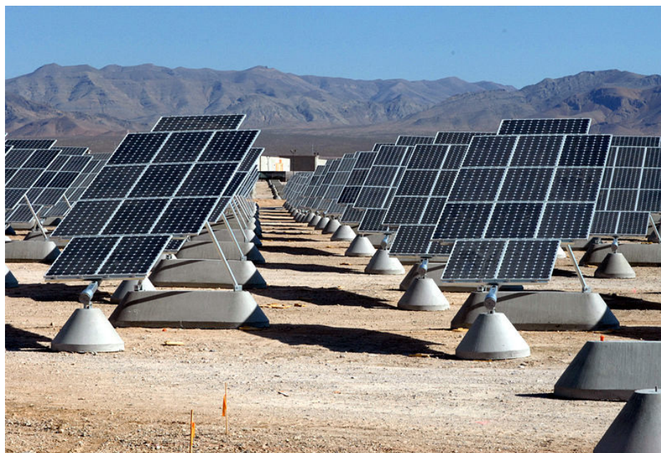
Photograph: Nellis Air Force Base, Nevada. The Solar Power Plant in Nevada is a 70,000 solar-panel installation, which at 14 megawatts, is the largest in North America.
