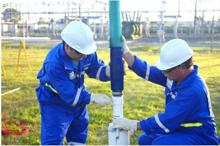
Schlumberger Westbay System is one commercial sampler option Uses packers to isolate zones, with independent pumping and sampling ports
