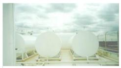
Figure 7-3: Shop-built containers elevated on saddles.
