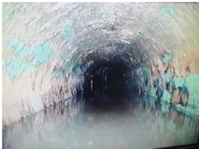
A screen capture from a sewer inspection video depicting evidence of discharges in the collection line, downstream of the Denali facility.
