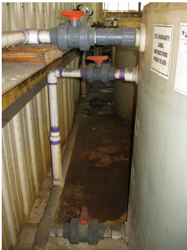
Pipes and valves located behind the nital etch tanks plumbed to a roof storm drain which was connected to a combined sanitary sewer.
