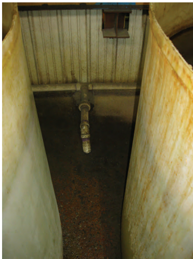
The location where Brad Foot Gear Works cut the concrete floor and installed piping to connect the nital etch tank drains to the combined sewer.
