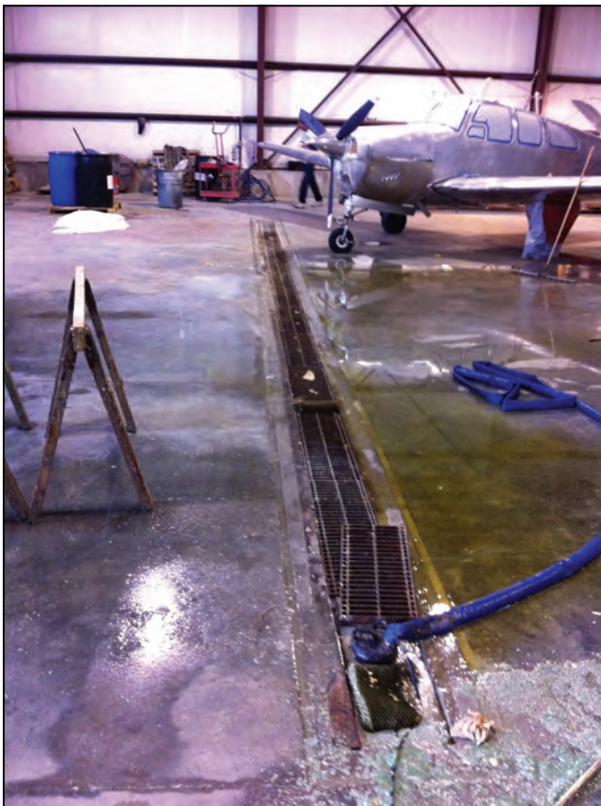
Gold Metal Paint Co. stripper hangar showing methylene chloride stripper waste drain.
