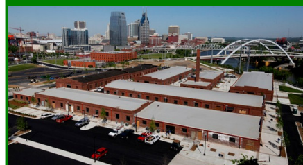
AFTER: Trolley barns rehabilitated to office and retail spaces
