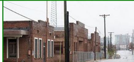
BEFORE: Historic Trolley barns created from the Works Progress Administration
