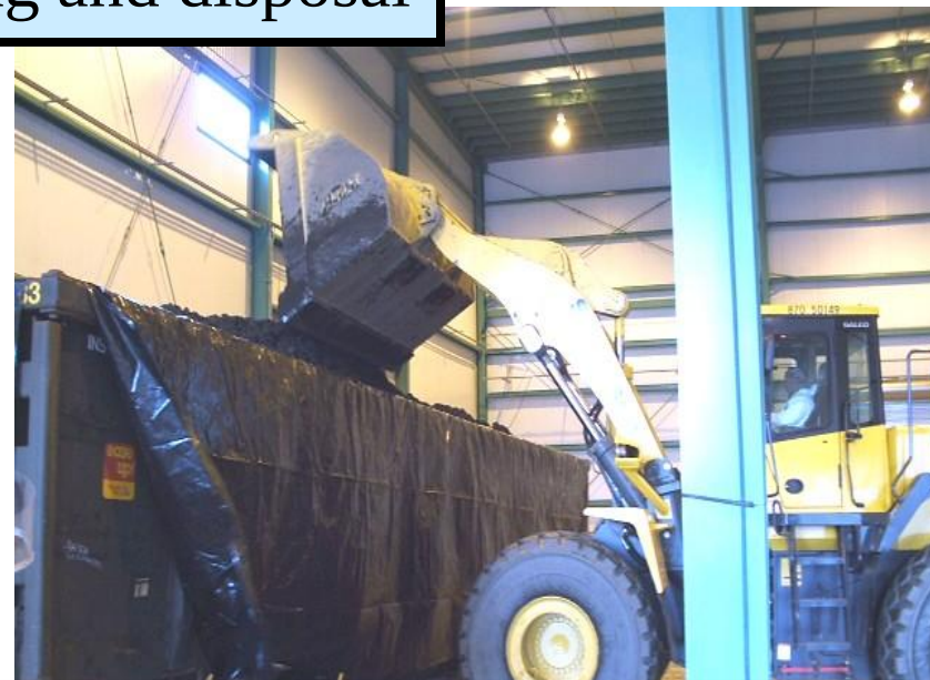
Step 4. Loading to rail for offsite disposal
