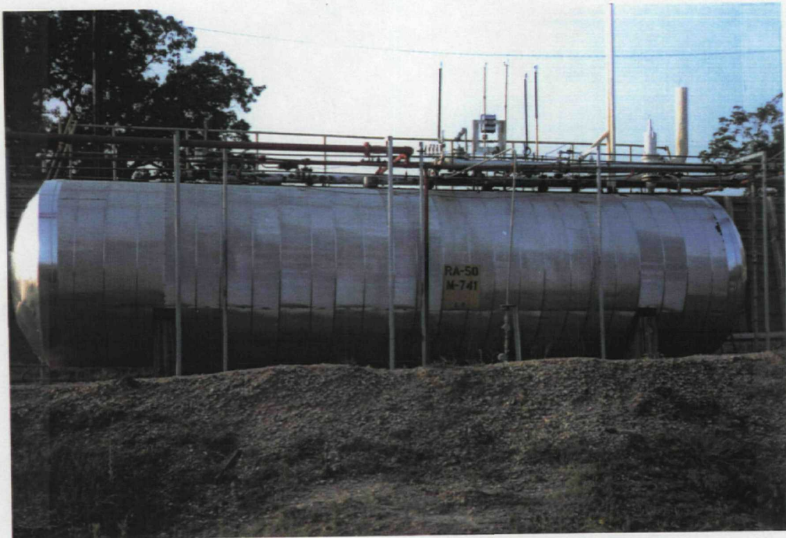
Photo # 17 Roll # 1 Frame #: 18 Date: 6/25/92 Subject: The E-0 Tank (Ethylene Oxide) located in the northeast portion of site property.
