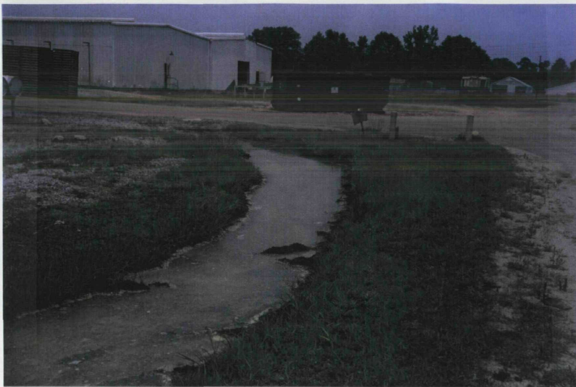
Photo № 27 Roll № 2 Frame №: 6 Date: 6/25/92 Subject: North view of drainage ditch which lies along eastern portion of site property. Location of HI-SD-04.
