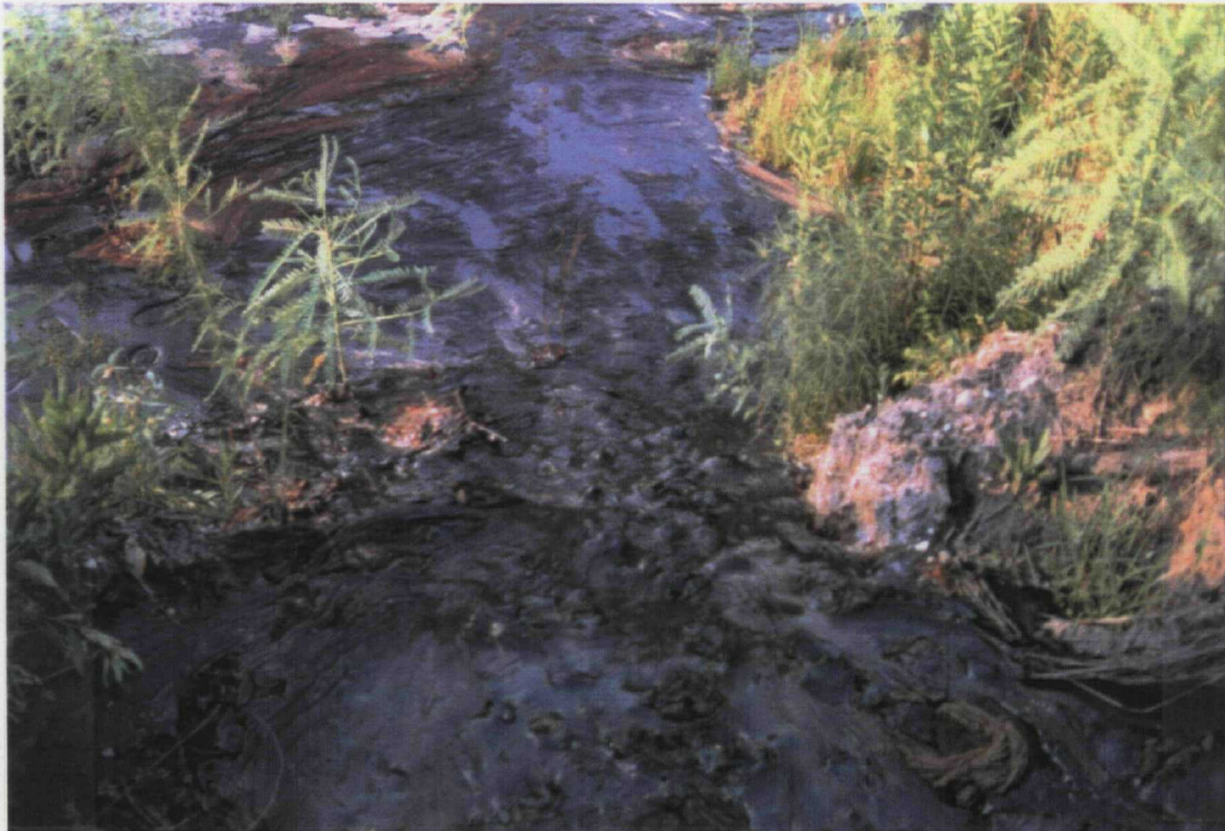
Photo № 14 Roll № 1 Frame №: 15 Date: 6/25/92 Subject: A dike breach in the sludge pits located near the E-0 tank, northeast corner of site property.
