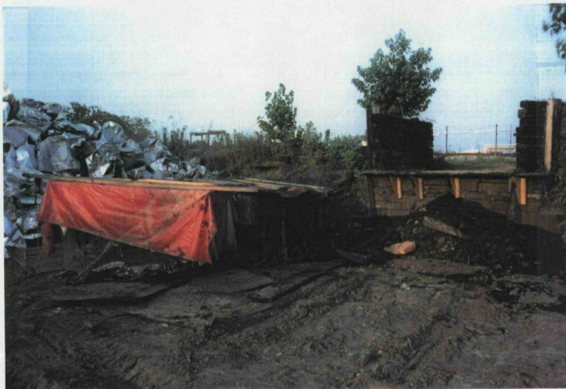
Photo № 22 Roll № 1 Frame №: 24 Date: 6/25/92 Subject: Dumpster on left (covered with a tarp) which has been filled off the unloading dock. Note: Dumpster was removed, area was "clean" during the second site visit in August 1992.
