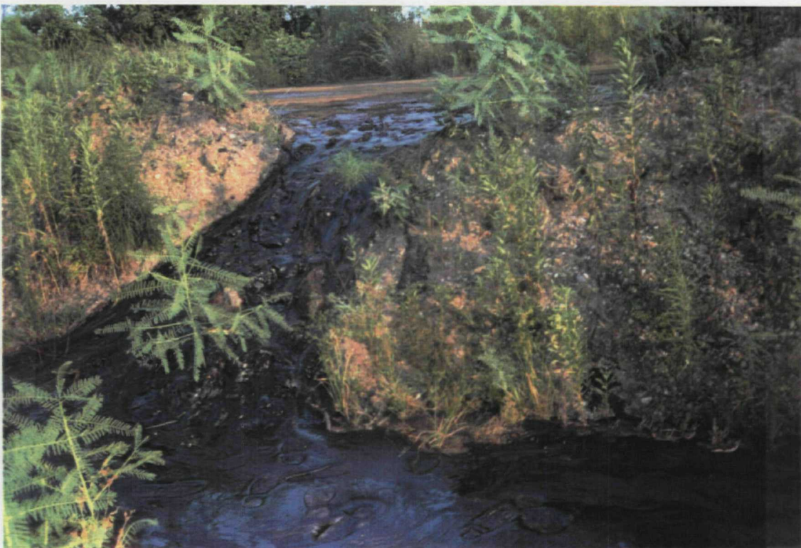
Photo № 19 Roll № 1 Frame №: 20 Date: 6/25/92 Subject: Sludge flow through a breach in the containing dike. Near the E-0 tank.
