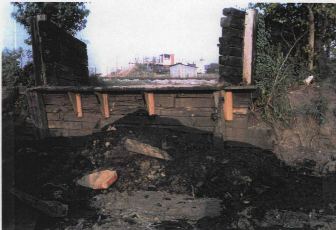
Photo № 21 Roll № 1 Frame №: 23 Date: 6/25/92 Subject: The unloading dock located near the drum recycling area. Location of HI-SS-02. Notice the stained soil and stressed vegetation.
