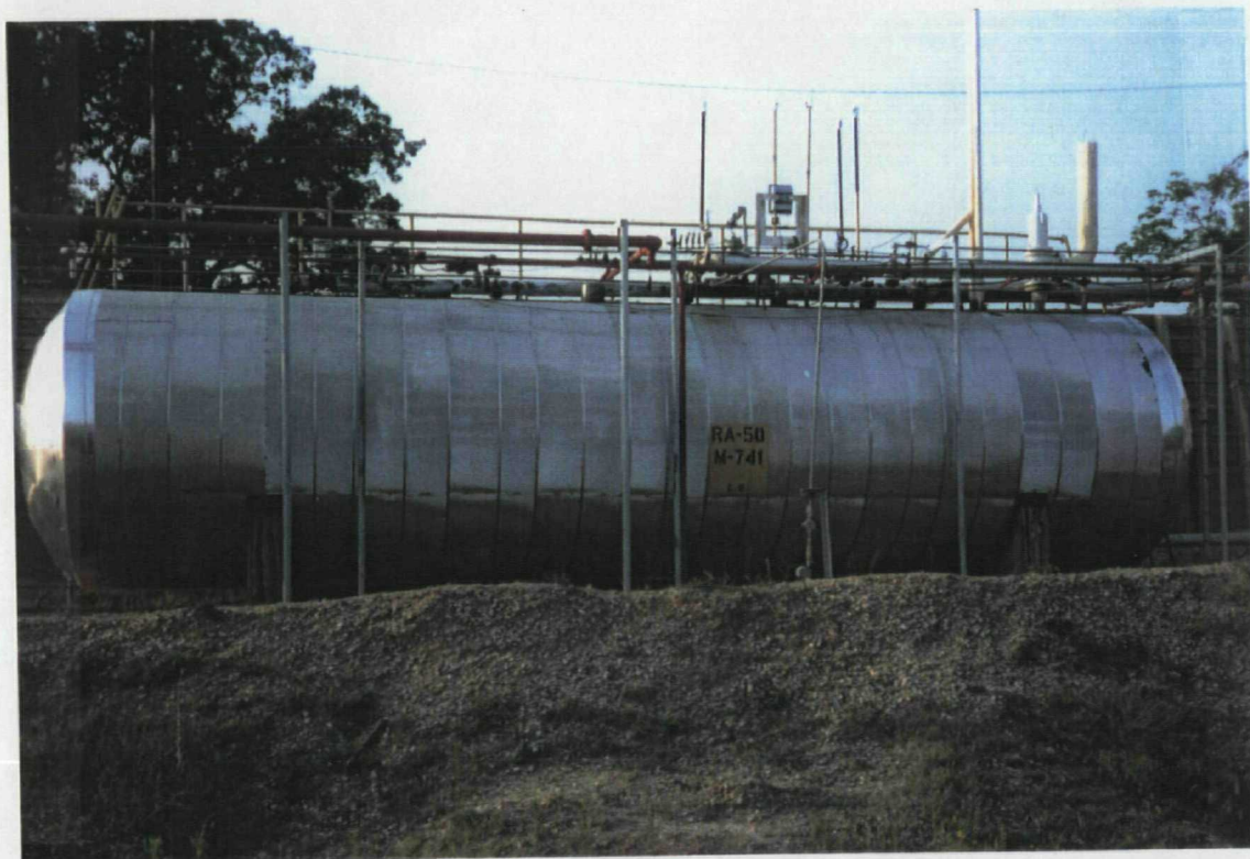
Photo № 17 Roll № 1 Frame №: 18 Date: 6/25/92 Subject: The E-0 Tank (Ethylene Oxide) located in the northeast portion of site property.
