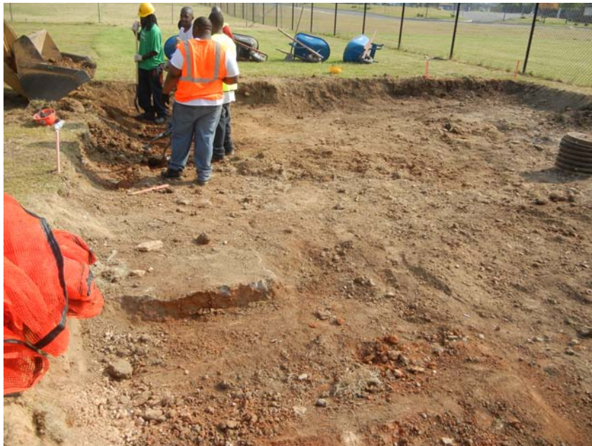
5. Concrete footing in area hand-excavated area over the retention unit.
