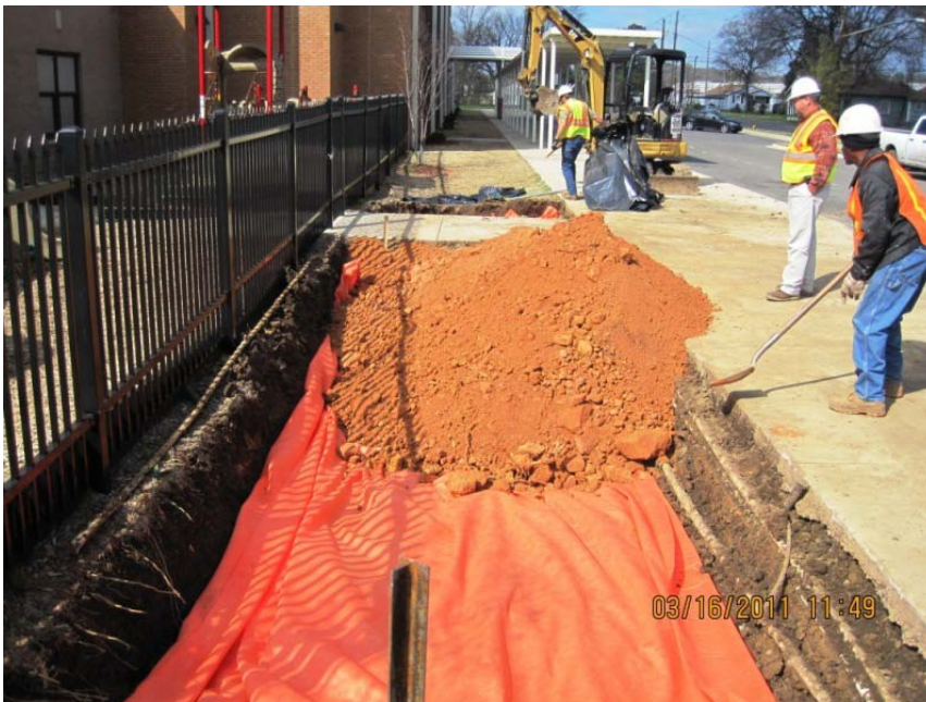
2. Clean fill being placed above geotextile fabric barrier in the excavation at the northern portion of the school.
