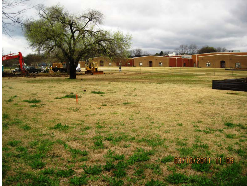
4. Pre-excitation at the southern area of Hudson school (north-east facing).
