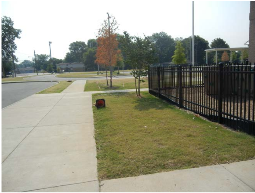
3. Post-excavation at the northern portion of Hudson school (East facing).
