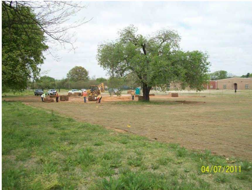
8. Post-excavation at southern area of Hudson school (north-east facing).
