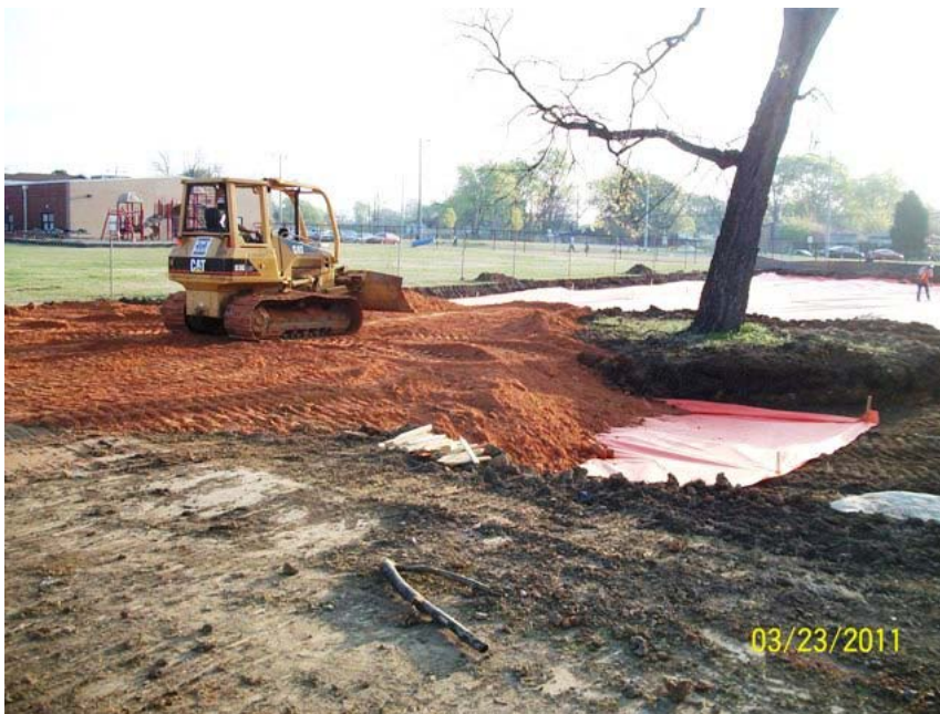
7. Clean fill being placed above geotextile fabric barrier in the southern area excavation.
