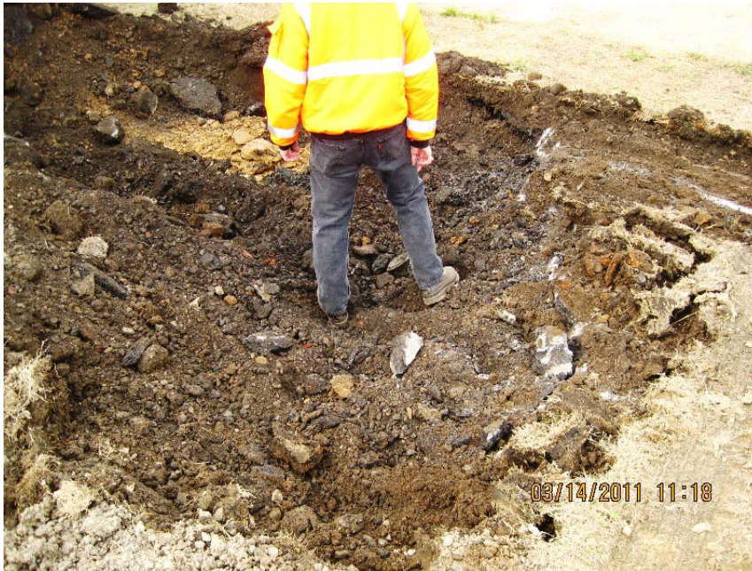
6. Asphalt debris uncovered in the northwestern portion of the larger southern excavation area.
