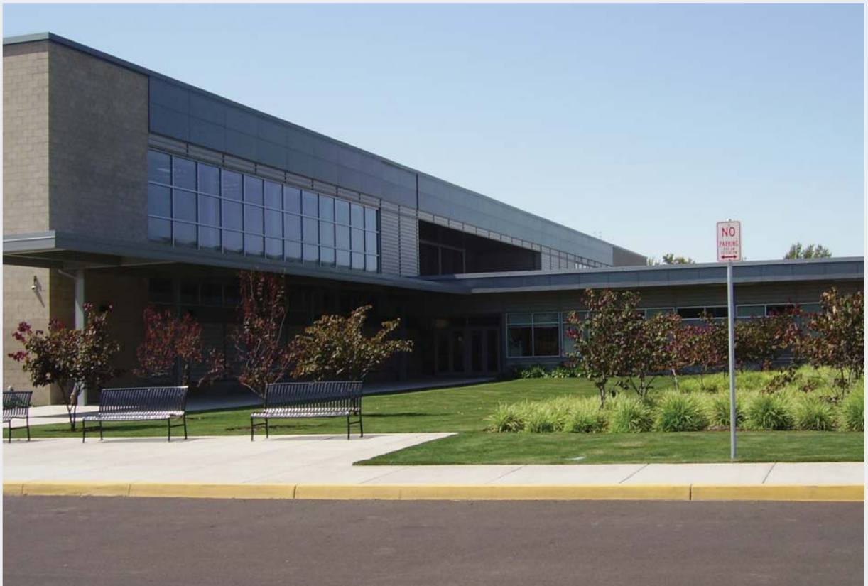
The LEED-certified Sue Buel Elementary School in McMinnville, Oregon
