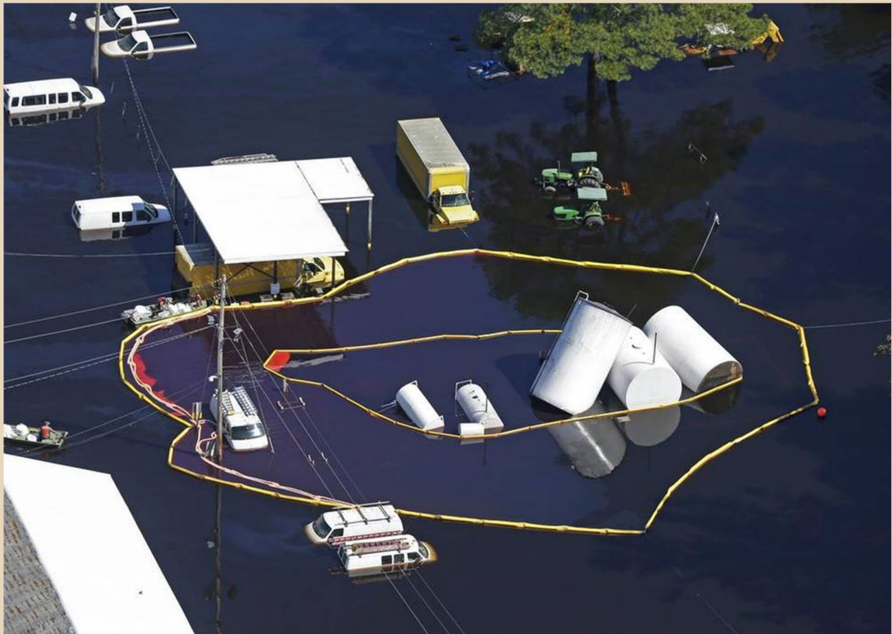
Facility with displaced ASTs, product release, and fuel containment – Hurricane Matthew, 2018. Credit: NCDEQ
