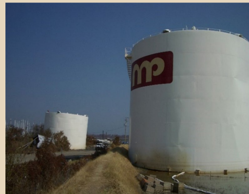
420,000-gallon tank floated out of a containment berm. Credit: NISTM
