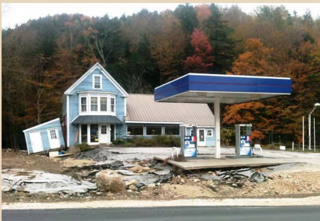
Blackie's General Store - Soil erosion and scour from Ottaquehee River flooding. Tropical Storm Irene - August 2011. Credit: New England Interstate Water Pollution Control Commission
