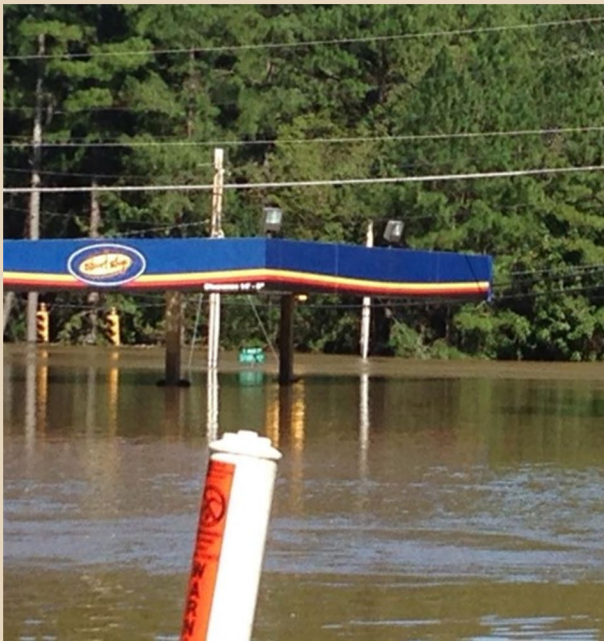
Flooded gas station. Hurricane Matthew, 2016 Credit: NCDEQ
