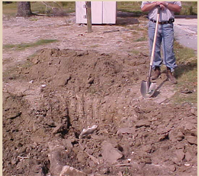
Digging to locate USTs after Hurricane Katrina. Credit: EPA
