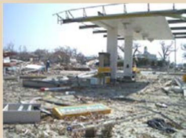
Gas station "debris field" after a flood. Credit: EPA
