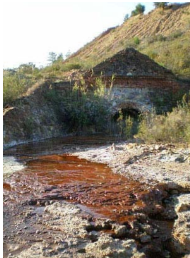
Figure 2: Roman Portal with Acid Rock Drainage – Spain
