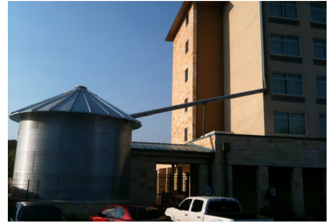
Figure 22: Nearby Hotel with Stormwater Capture Cistern
