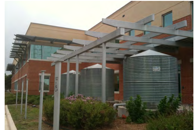
Figure 23: San Antonio Municipal Building with Air Conditioning Condensate Reuse
