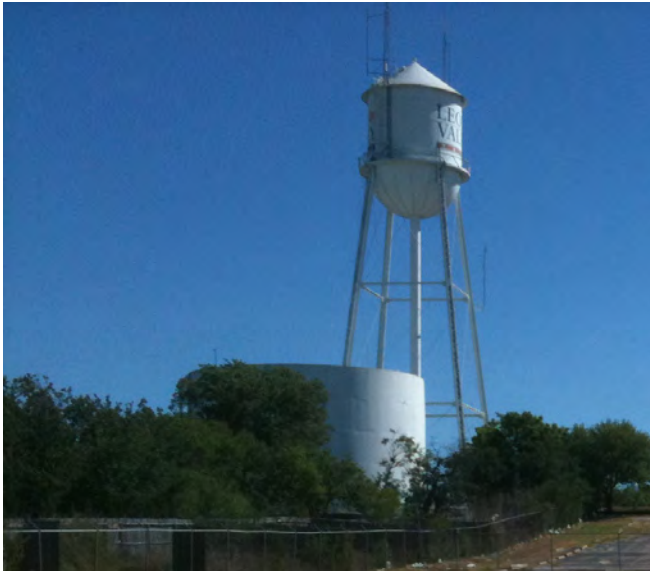
Figure 34: Leon Valley Water Tower as Seen from Site
