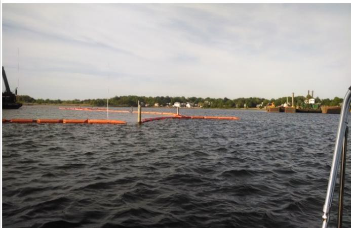
Silt curtain reattached to the pylon
