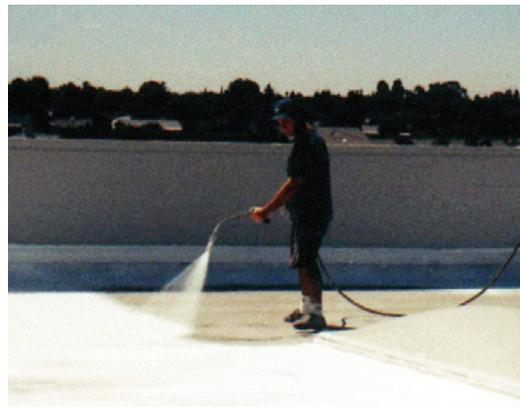
Cool coating being sprayed onto a rooftop.
