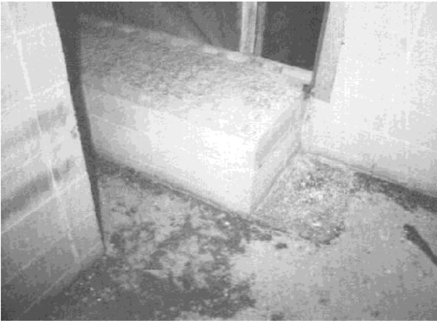
*An initial walkthrough may uncover problems such as this unsanitary condition in the HVAC system. Bird droppings have collected in an air supply plenum near an outdoor air intake that was not protected by a birdscreen.*
