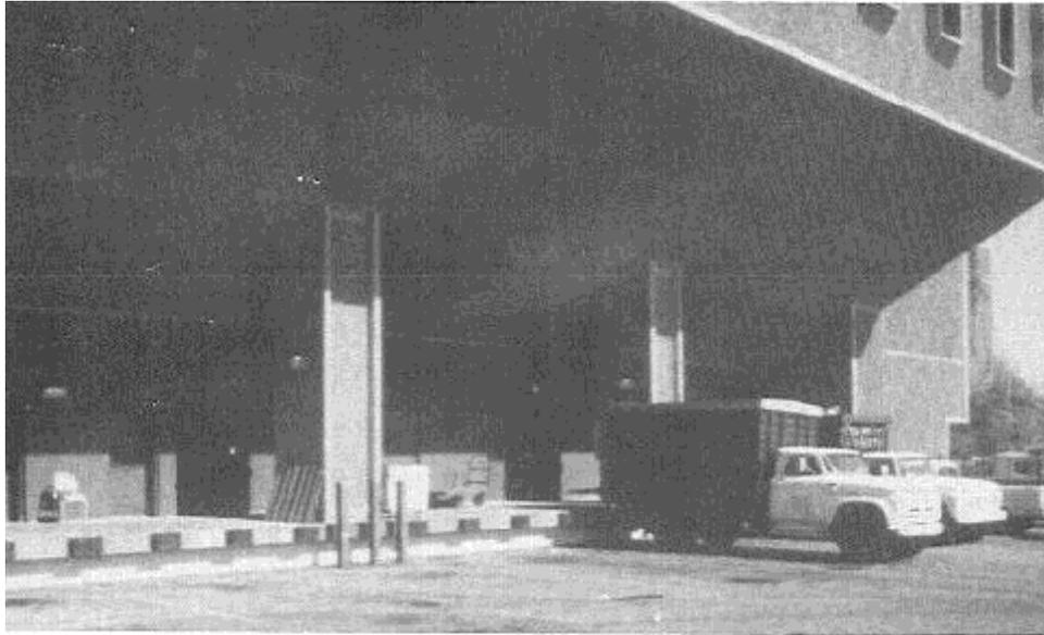
*Exhaust fumes are drawn into this building's outdoor air intake when trucks are idling at the nearby loading dock. Tools such as the Occupant Diary and Log of Activities and System Operation can help to identify intermittent pollutant sources such as this one.*
