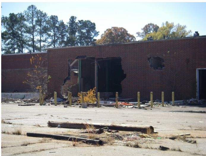
Rear view of Haynsworth Mill where steel removal operations occurred, causing asbestos to become disturbed.
