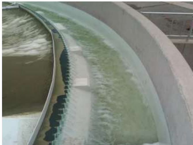
Figure 7-9 Dissolved air flotation thickening (DAFT) at the Stockton, California wastewater treatment facility (Parlin, pers. comm. 2010).
