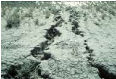
Figure 4-1 An example of eroded dike slopes.
