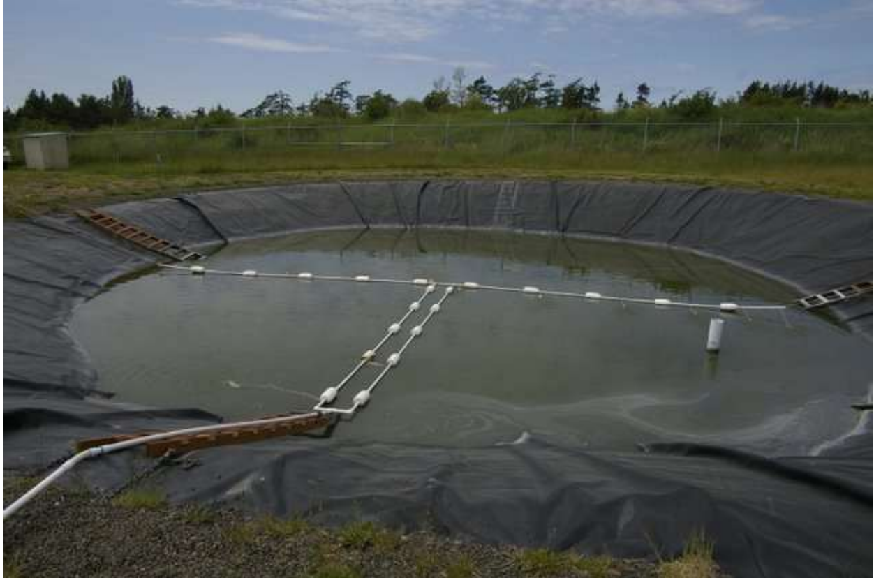
Figure 5-21. Fisherman Bay, Washington. Anaerobic cell with recirculation manifold using an aerated cap of polishing cell effluent to provide odor control.
