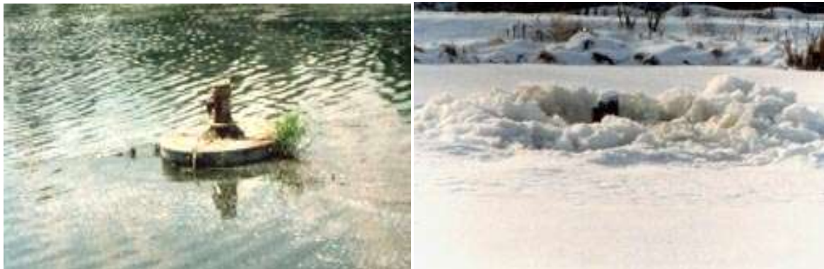
Figure 3-3. Floating aerators in summer and winter operation.
