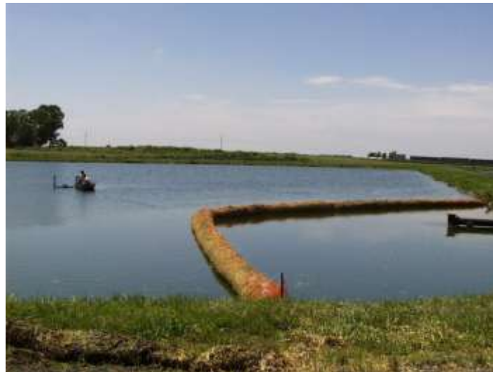
Figure 7-11. A barley straw boom in cell 3, New Baden, Illinois wastewater pond system.
