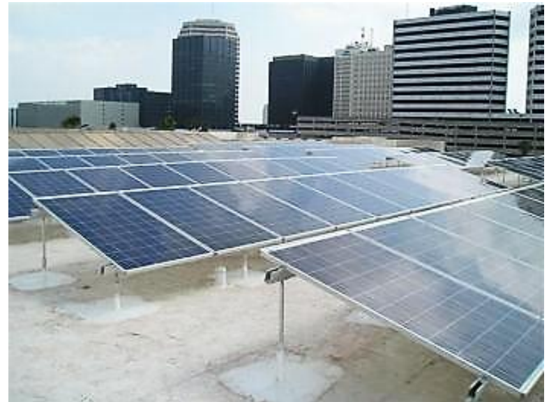
25KW PV System
