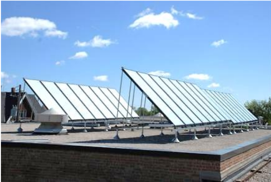
Solar Water Heating System (84) - 4' x 10' collectors = 3360 ft 2
