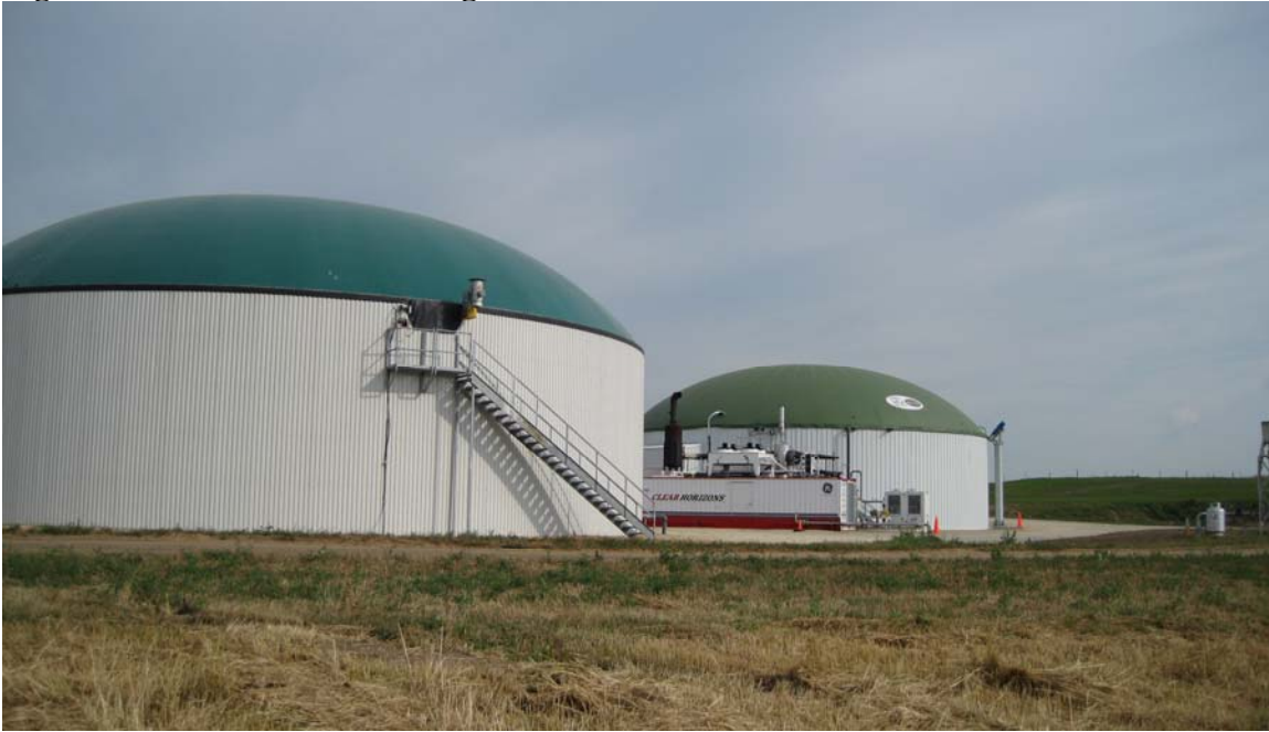
Figure 12 – Crave Brothers Digesters
