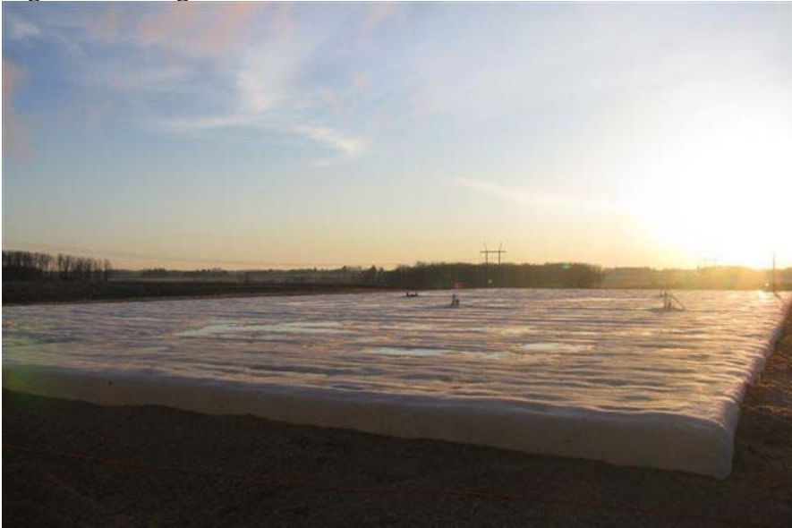
Photo courtesy of Norm-E-Lane
