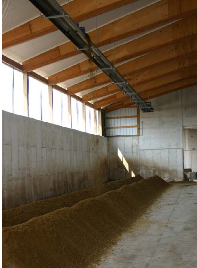
Figure 51 – Separated Solids Conveyor and Storage
