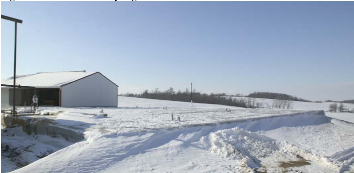
Figure 8 – Clover Hill Dairy Digester
