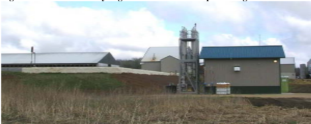
Figure 21 – Emerald Dairy Digester and Gas Cleanup Building
