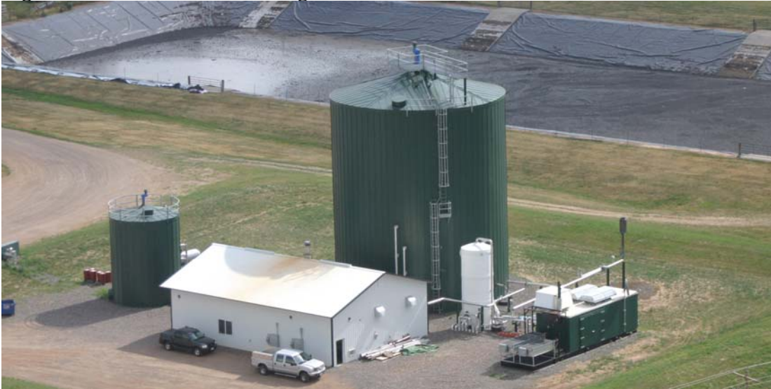
Figure 40 – Norswiss Farms Digester
