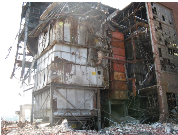
Stripped boiler from powerhouse of the facility
