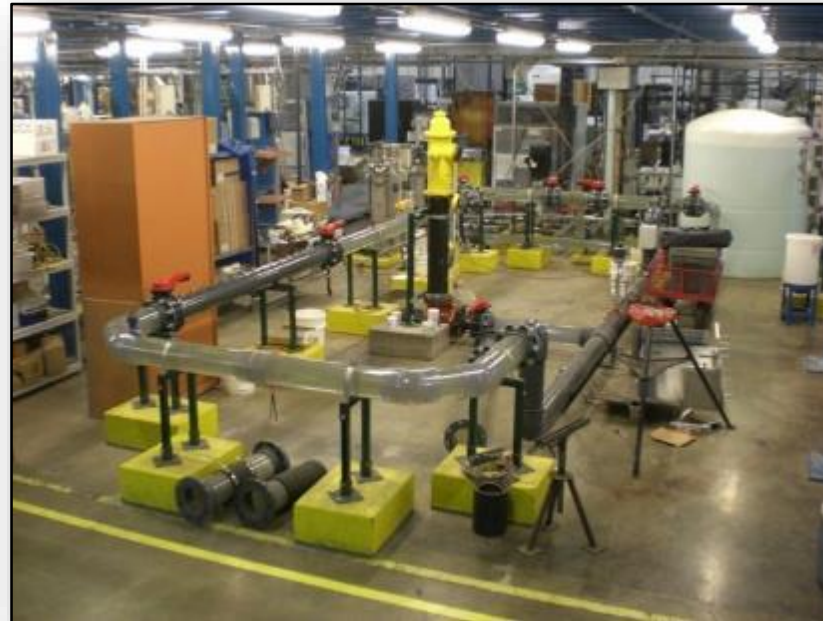
Test and Evaluation Facility where the on-line monitors and pilot decon approaches are assessed
