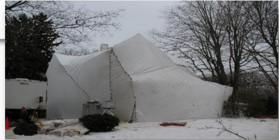
House contaminated with anthrax is tented in preparation for fumigation
