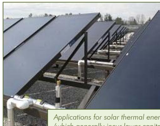
*Applications for solar thermal energy (which generally incur lower capital costs than photovoltaic systems) include heating, cooling, ventilation, hot water heating, or process heating.*
