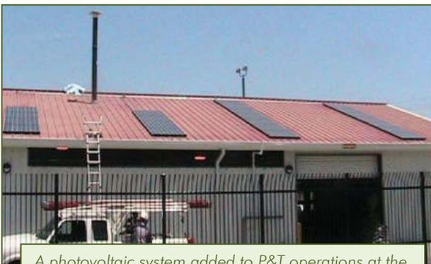
*A photovoltaic system added to P&T operations at the Pemaco Superfund Site in Maywood, CA, contributes 5,900 kWh of electricity each year to high-vacuum dual-phase extraction of groundwater.*
