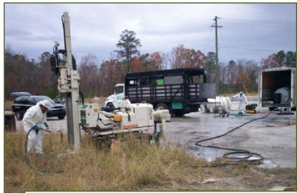
*Integrated planning of bioremediation activities at Marine Corps Base Camp Lejeune enabled injections of emulsified vegetable oil and sodium lactate in four borings to be completed within only one week, which reduced field redeployment and associated fuel use.*
