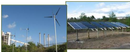
Use of this direct drive electricity system avoids the need for storage batteries, consequently lowering the project's capital and maintenance costs and avoiding battery disposal. Capital costs (excluding wells and pumps) totaled approximately \$50,000, or about 50% of the expected cost for grid connection. More savings were gained through federal tax credits received by the site owner. Each day, the system recovers approximately 113 gallons of free product and 25,000 gallons of groundwater.
