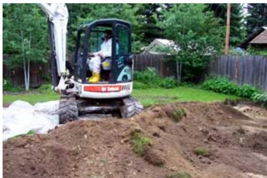
Exterior removal of contaminated soil from a residential area. (EPA photo)
