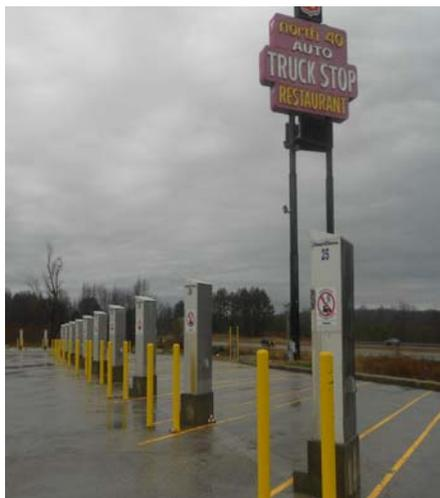
Truck stop electrification equipment at a truck stop in Holladay, Tennessee. (EPA OIG photo)
