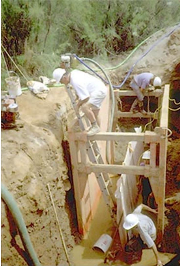
**Figure 5.1.** Trench box used to protect workers during installation of the PRBs at Fry Canyon, Utah.
