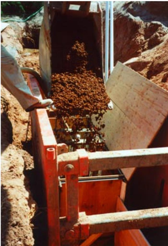
**Figure 5.2.** Placement of AFO barrier material into the gate structure of the permeable reactive barrier, Fry Canyon, Utah.
