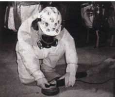
Sold by C.S. Unitec, Inc., the Lightweight Concrete Grinder is electrically powered. When used in a circular motion, it rapidly grinds concrete surfaces 1.5 to 3 millimeters deep. A dust collection shroud can is designed to attach to the vacuum hose of
