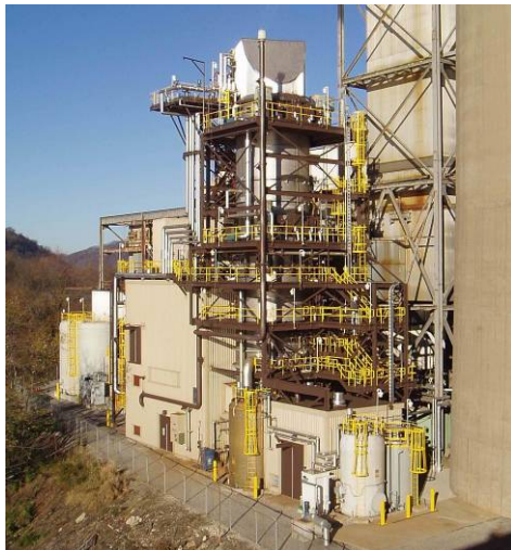
50 MW ECO pilot
