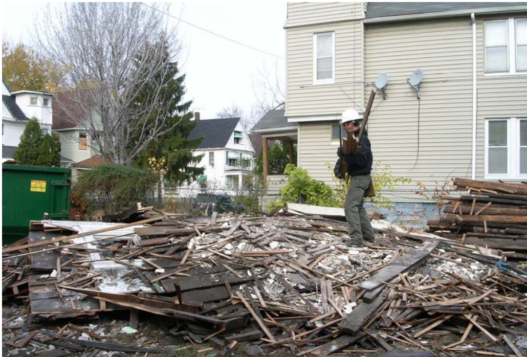
Photo 8 – Cleveland Deconstruction Initiative – Hand Dismantling
