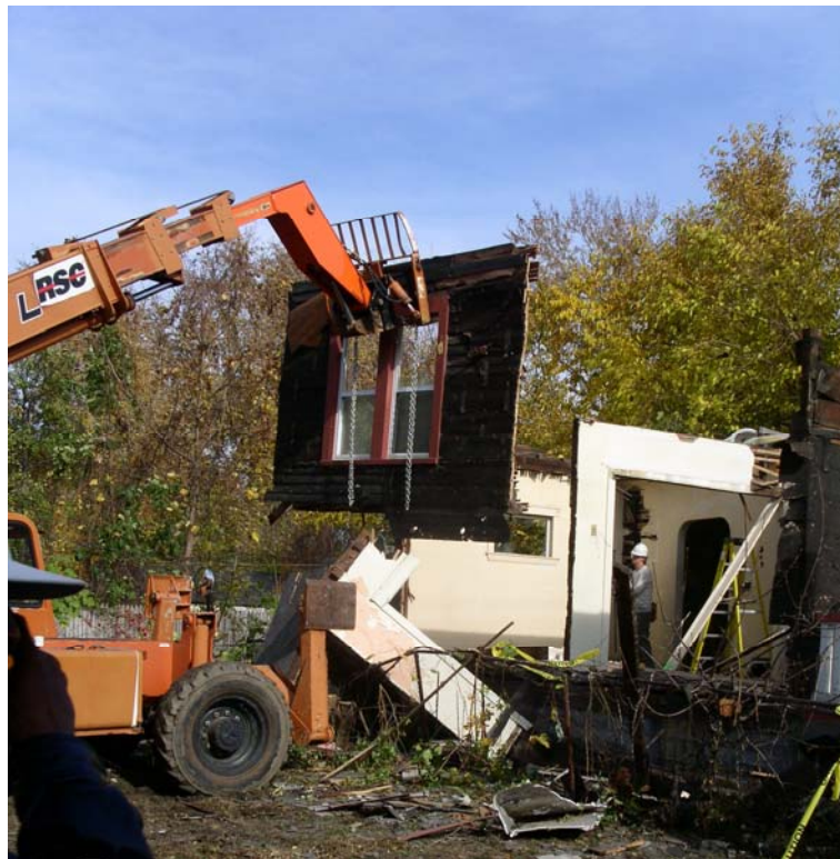
Photo 2 – Cleveland Deconstruction Initiative – Removal of House Panel
