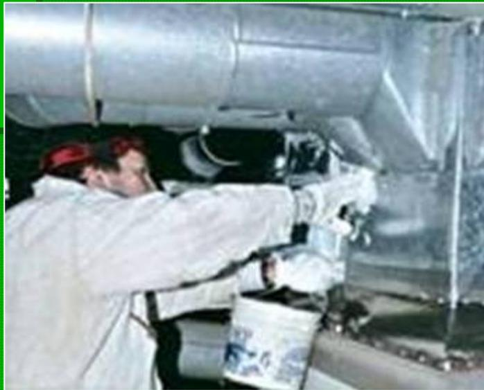
Critical Duct Sealing directly above furnace where majority of heat escapes from ducts
