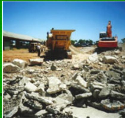
Crushed concrete as aggregate in new concrete
