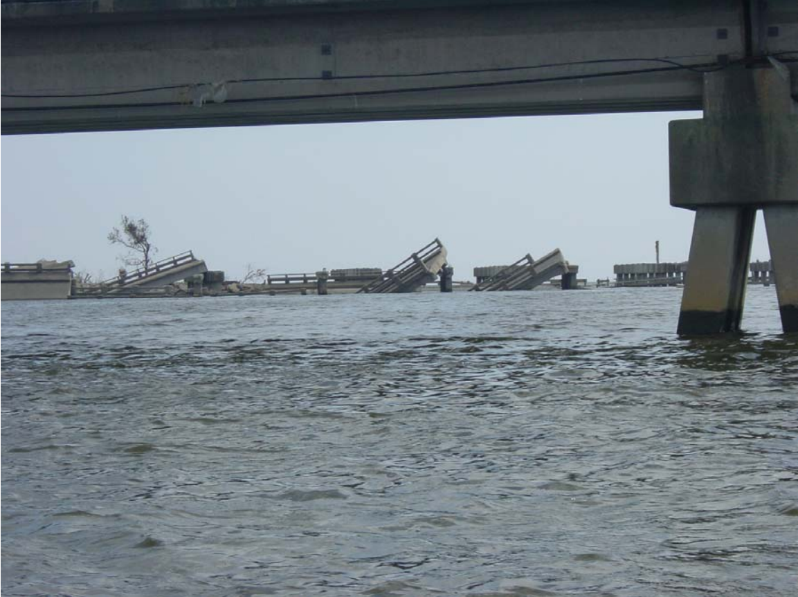
Figure 8, Back Bay of Biloxi @ Highway 90
