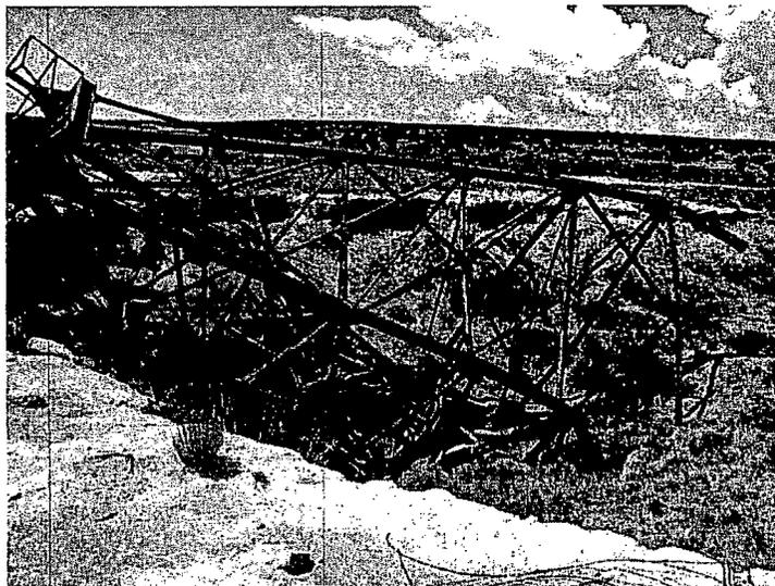
P1: Spencer Mine headframe collapsed into shaft due to arroyo capture and undercutting
