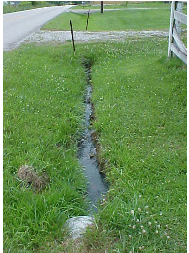
Straight Pipe Drainage: Preston, KY
