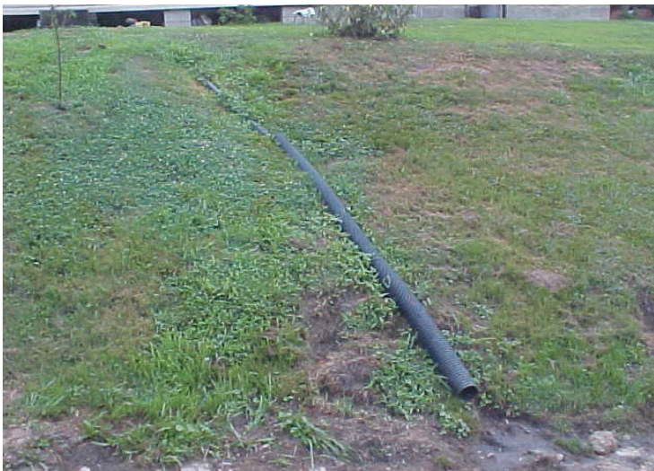
Straight Pipe: Martin County, KY
