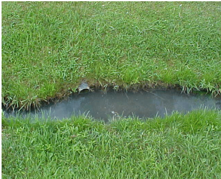
Septic drainage: Preston, KY
