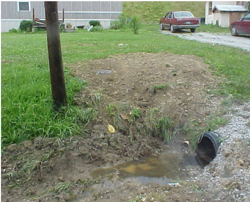
Straight Pipe:Martin County, KY
