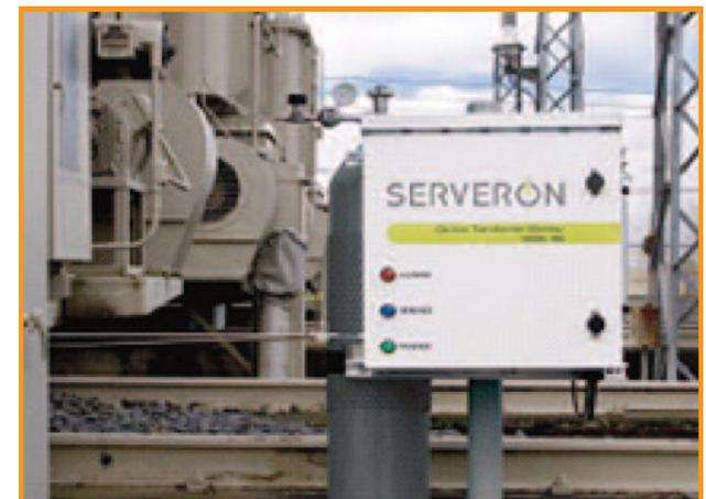
CMS' online transformer monitoring system, which monitors dissolved gases in transformer oil to protect against catastrophic transformer failure.
