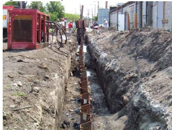
**Figure 7. Horizontal Electrode Installation**
