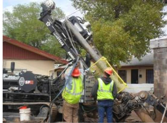
**Figure 6. Sheet pile Electrode Installation**
