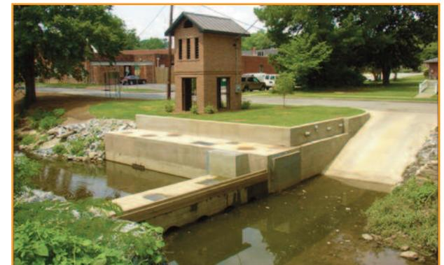
WWETCO Compressed Media Filter and Flow Controls with ultraviolet disinfection for Weracoba Creek stormwater treatment in Columbus, Georgia
