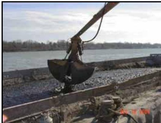
controls and careful operator practices were used to prevent removed sediment from being released into the river channel. The primary control was a “spill prevention plate,” which consisted of a steel plate that overlapped the transport barge and the silt curtain and lead back to the dredge plant. This plate was welded to 6 of the steel pipe pilings that
