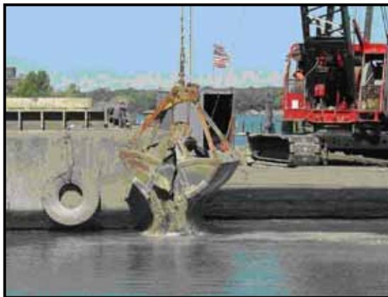
surface of the water to achieve a greater rate of dispersion and to reduce mounding. The cover materials were shuttled from the north end of the lagoon by hopper barge and tugboat, and the progression of cover material was from south to north.
