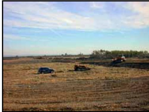
Dike construction material was originally to be obtained from within Cell 5, in the borrow area shown on the USACE drawings. This material was inappropriate, due to its water content and composition, therefore, material was conveyed from the offloading area to the cross dike location via 35-ton off-road articulated dump trucks.
