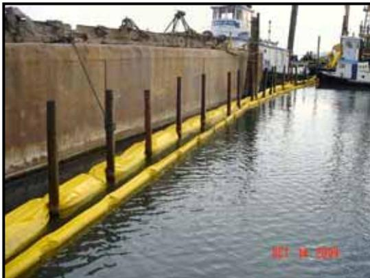
A 12-inch harbor boom was placed along the inner perimeter of the turbidity curtain to provide added containment of any potential oil sheen. Sorbent boom was also maintained directly inside the harbor boom to provide a secondary level of containment for potential oil sheen. Emergency oil spill containment equipment and materials were maintained
