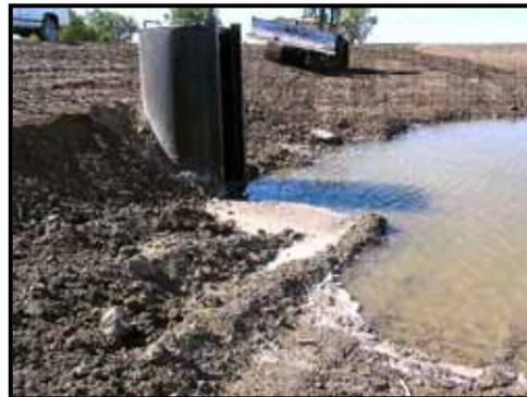
The soil was placed in layers not more than 12 inches in loose thickness, and each layer was compacted by a minimum of 3 passes of the D6 LPG dozer. Woven fabric liner of polyethylene geotextile was installed along the interior slope of the existing perimeter dike to confine the solidified dredged material and to prevent any seepage through the dike wall into Lake Erie or the Pointe Mouillee Wildlife Refuge. Inspections were made
