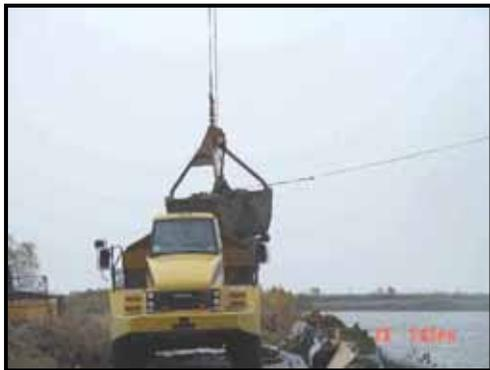
Dredged sediment from the Black Lagoon was received at the transfer/offloading area of the CDF. The tug and barges entered the CDF through the Southeast Interior Channel, where a smaller harbor tugboat (e.g., 35-foot, 300-horsepower) was used to maneuver the barges and place them at the transfer site. The barges
