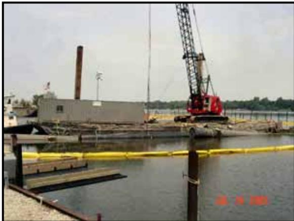
*Additional Environmental Controls.* An additional turbidity curtain was strategically placed perpendicular to the inner permeable curtain (i.e., east to west). The curtains were bolted together from surface to sediment and prevented recontamination as each cell was completed. In addition to the turbidity curtains, a barrier consisting of 3 to 7
