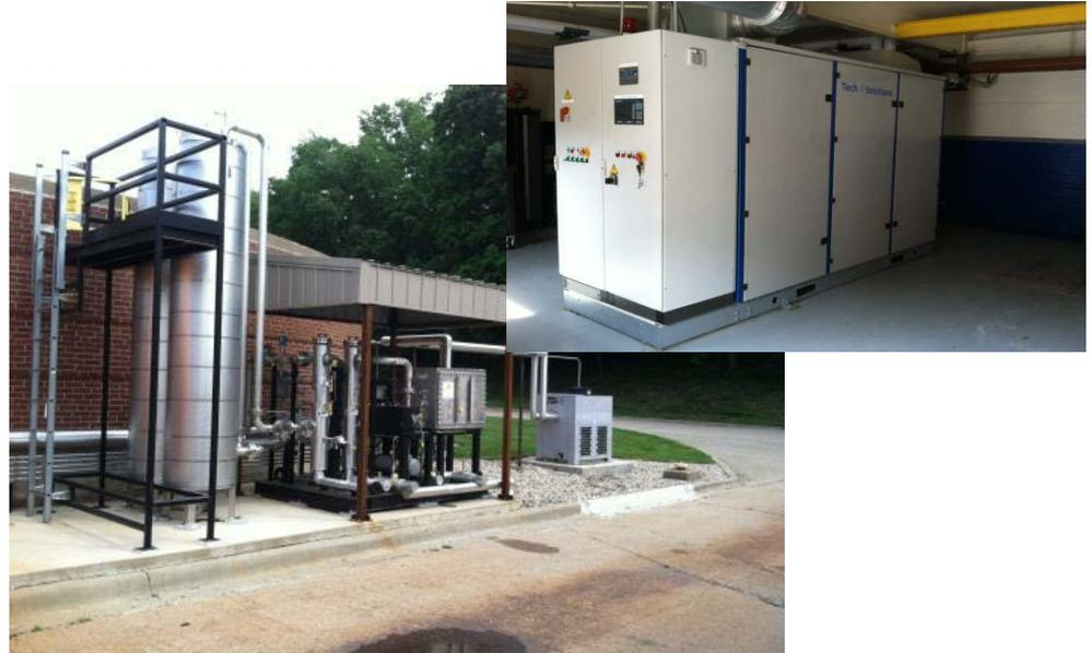
*Solids collected by the sewers from the residential, industrial, and commercial districts are separated from the accumulated solids. The separated solids [sludge] are pumped into anaerobic digesters that produce gas to fuel the engine.*
