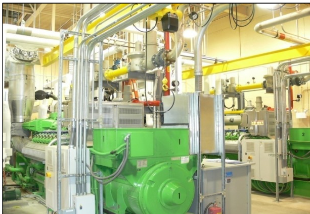
Internal Combustion Engine CHP System at Bergen County Utility Authority, Little Ferry, New Jersey
