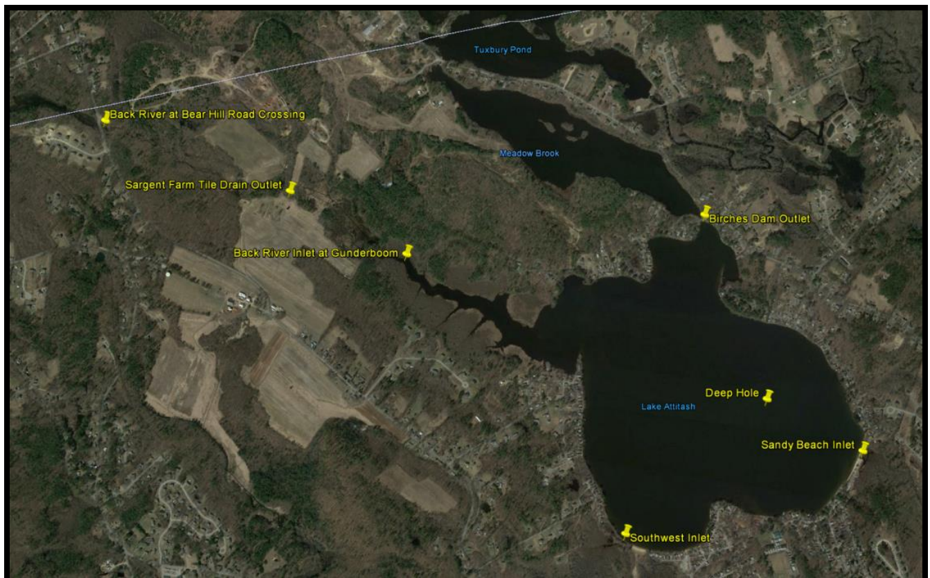
Figure 3-1: 2011 Dry weather sampling locations without stormwater outfalls.
