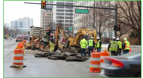
Figure 9: Infrastructure repair in Detroit, Michigan.
