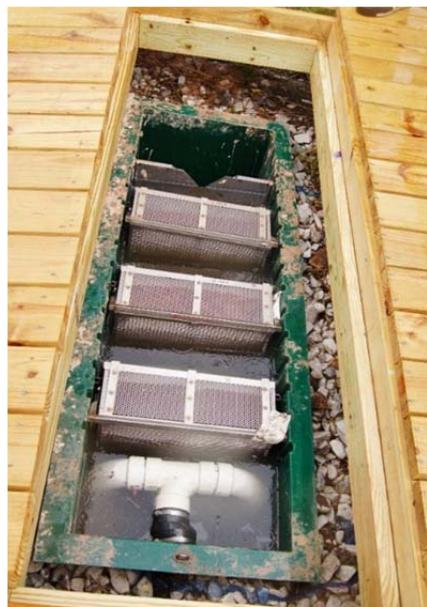
Exterior and interior views of the bark filter unit. The wooden platform acts as a cover to prevent tampering
