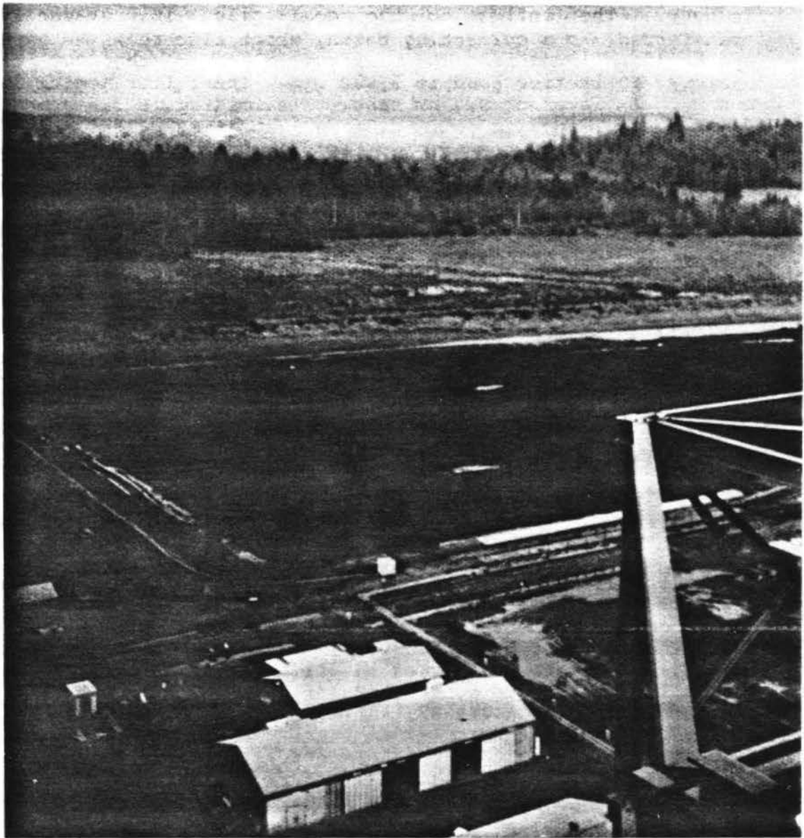
COAL PILE PLANT NO. 5305
