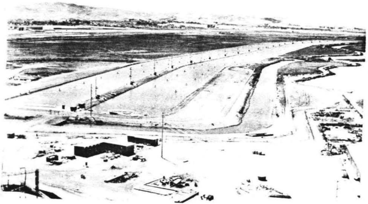
SPRAY CANAL PLANT NO. 0610 Figure B-VII-30
