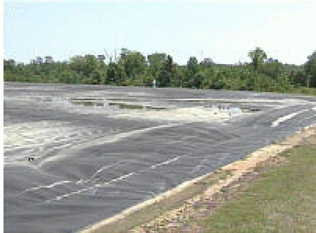
Some covered lagoons can also be converted into anaerobic digesters which rely upon a bacterial process to produce methane gas while decomposing organic wastes. The methane generated from the anaerobic digestion can be burned in an engine generator to produce electricity or in a boiler to produce heat. Digesting manure may reduce odor emission, fly production, and may help control some pathogens. CAFOs should be cautioned that digesters still require effluent holding.
