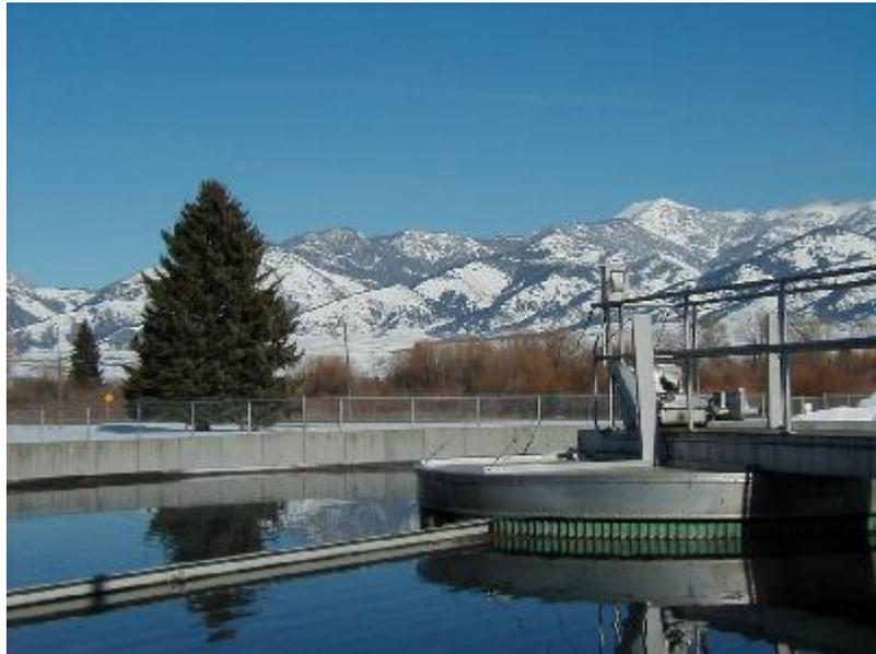
The project team's goal was to achieve interim compliance with new nutrient limits imposed by the Montana Department of Environmental Quality. To do this, the team decided to modify the existing activated sludge system so it would operate as a plug-flow process with phased nitrification and denitrification.
