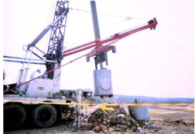
**Figure C-10. LFG Well Drilling.**
