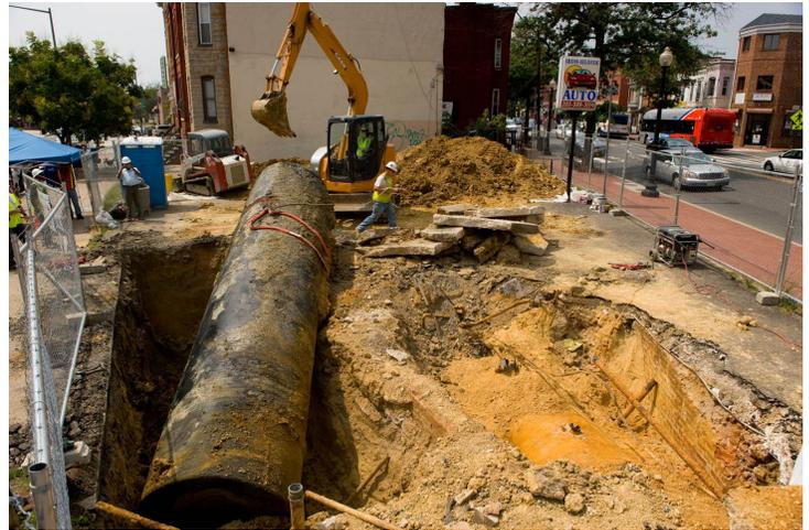
Figure 1: Underground Storage Tank Removal
