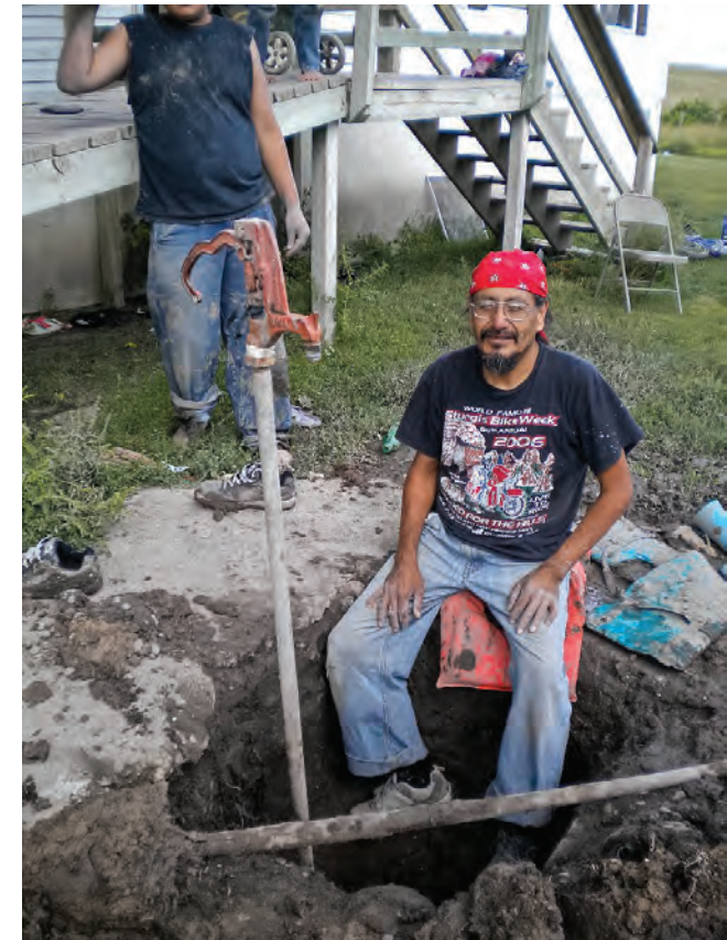
A local Pine River Reservation resident works on a pump to provide a house with well water.
