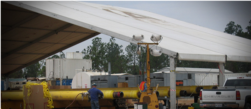
Example of Temporary Industrial Structure
