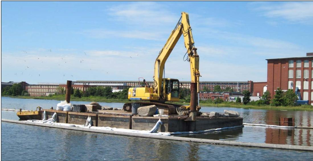
**Figure 8. Debris removal excavator and debris storage scow**
